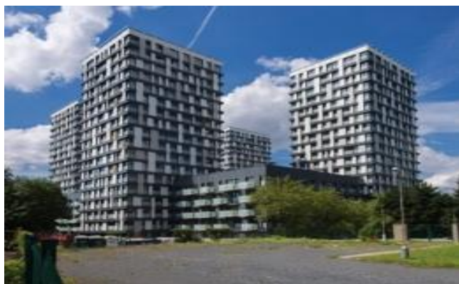
The Garden Towers ,Praha
